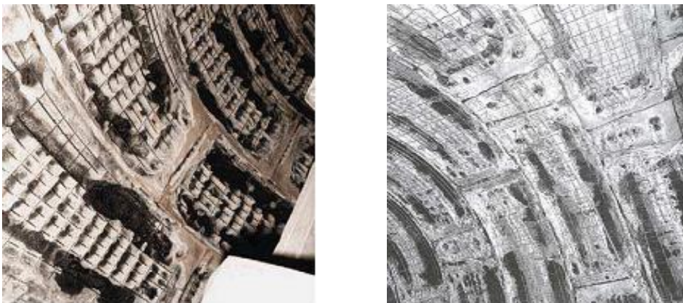
Figure 1. Fire damage in the English channel tunnel, 1996 (Mindeguia, 2009)
