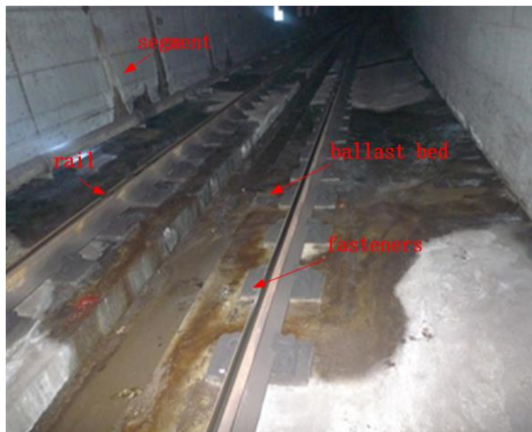
Figure 1. Metro ballast bed.
